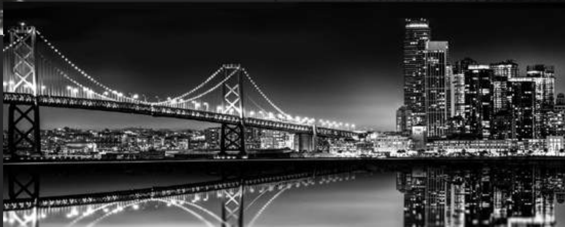
CA-12203 • ST485 • Bridge
